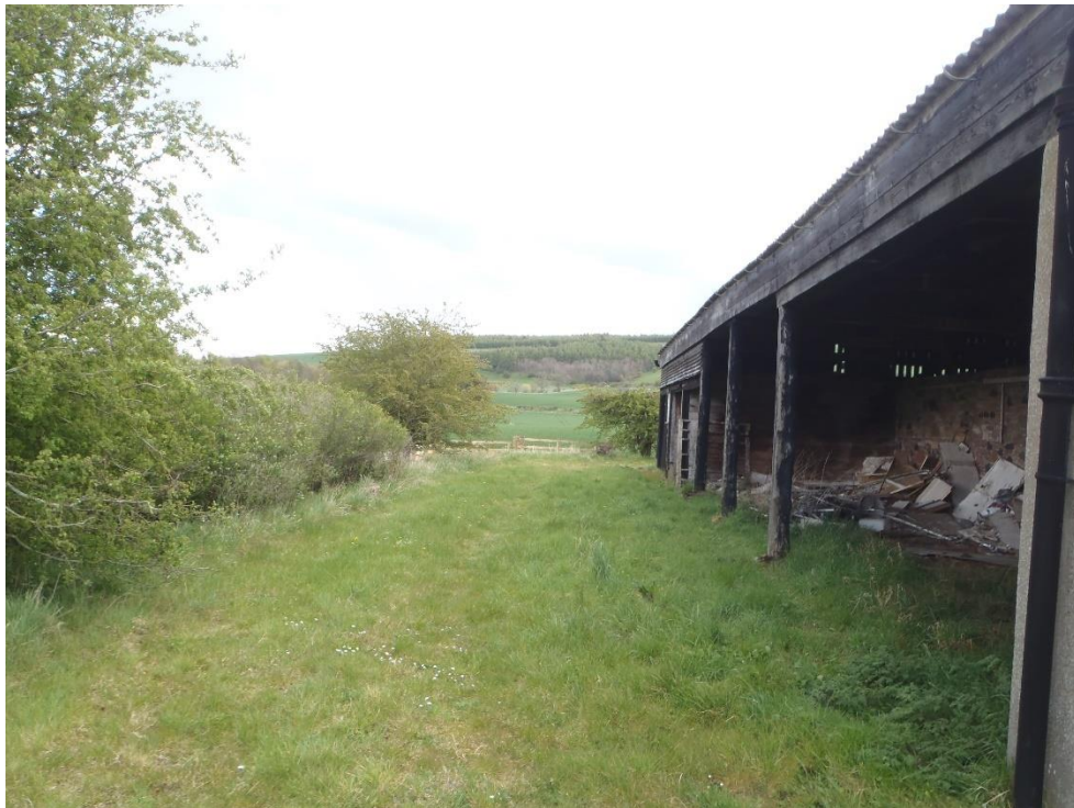
Photograph 3: showing a view of the grassland around the barn
