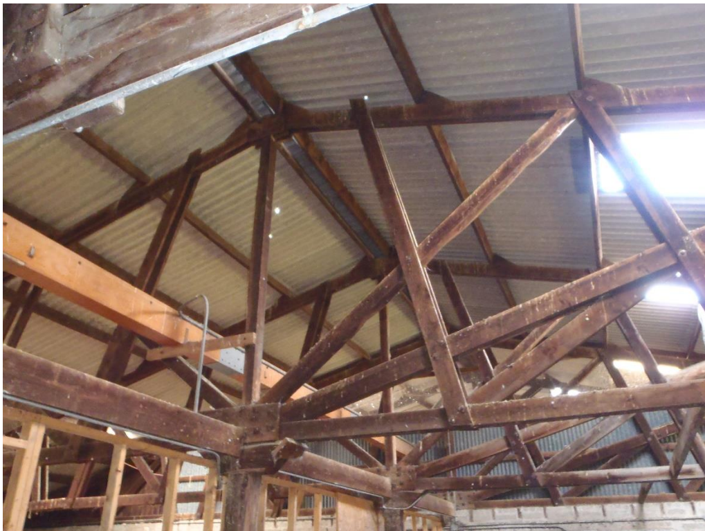
Photograph 7: Showing a view the barn roof
