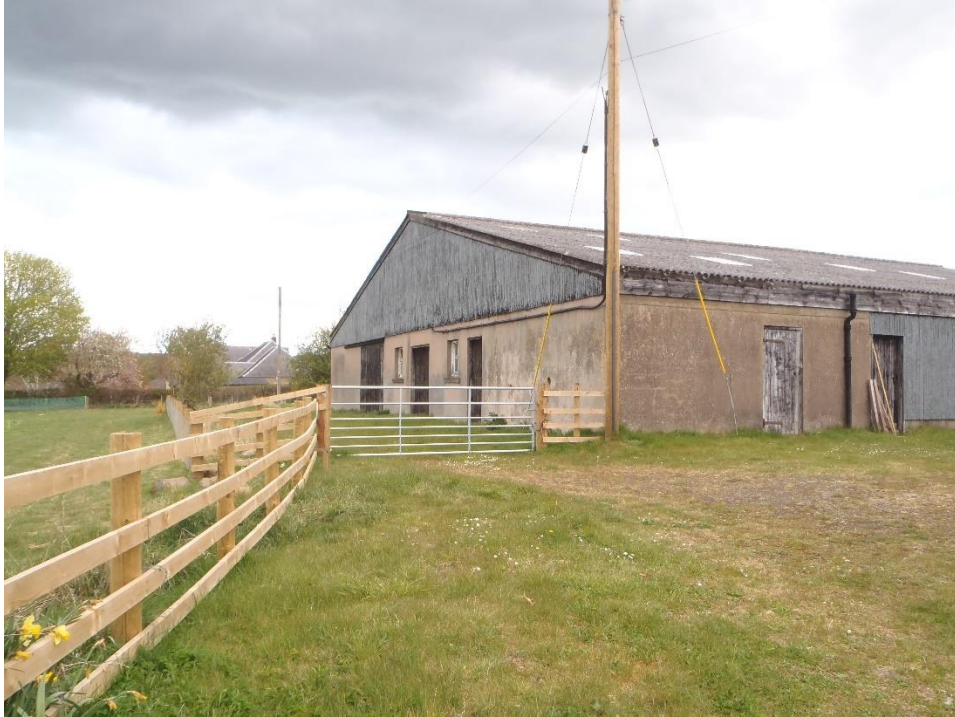
Photograph 2: showing a view of the site
