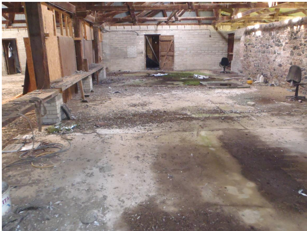
Photograph 6: Showing a view inside the barn
